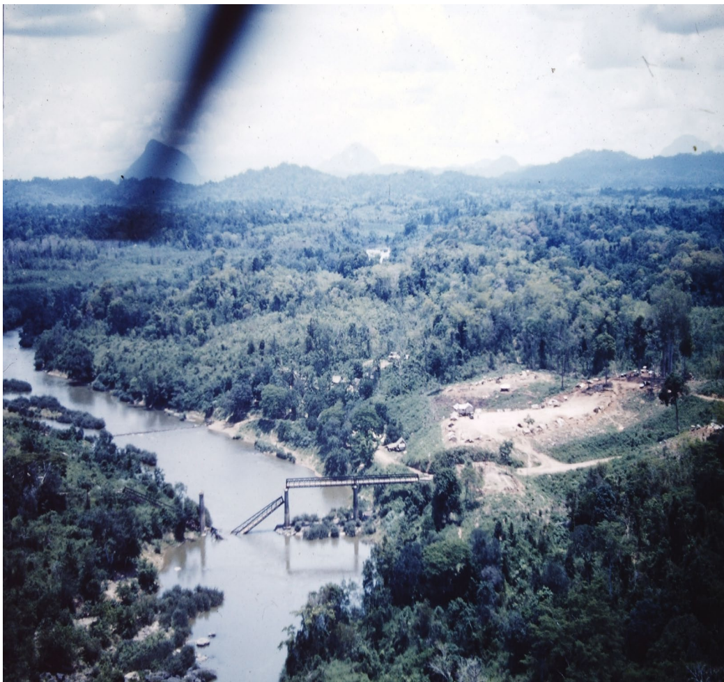
A broader view of the destroyed bridge over the Nam Lik at Ban Hin Heup leading to a government camp. A smaller pontoon bridge had been erected to a hamlet upriver from the downed structure.
