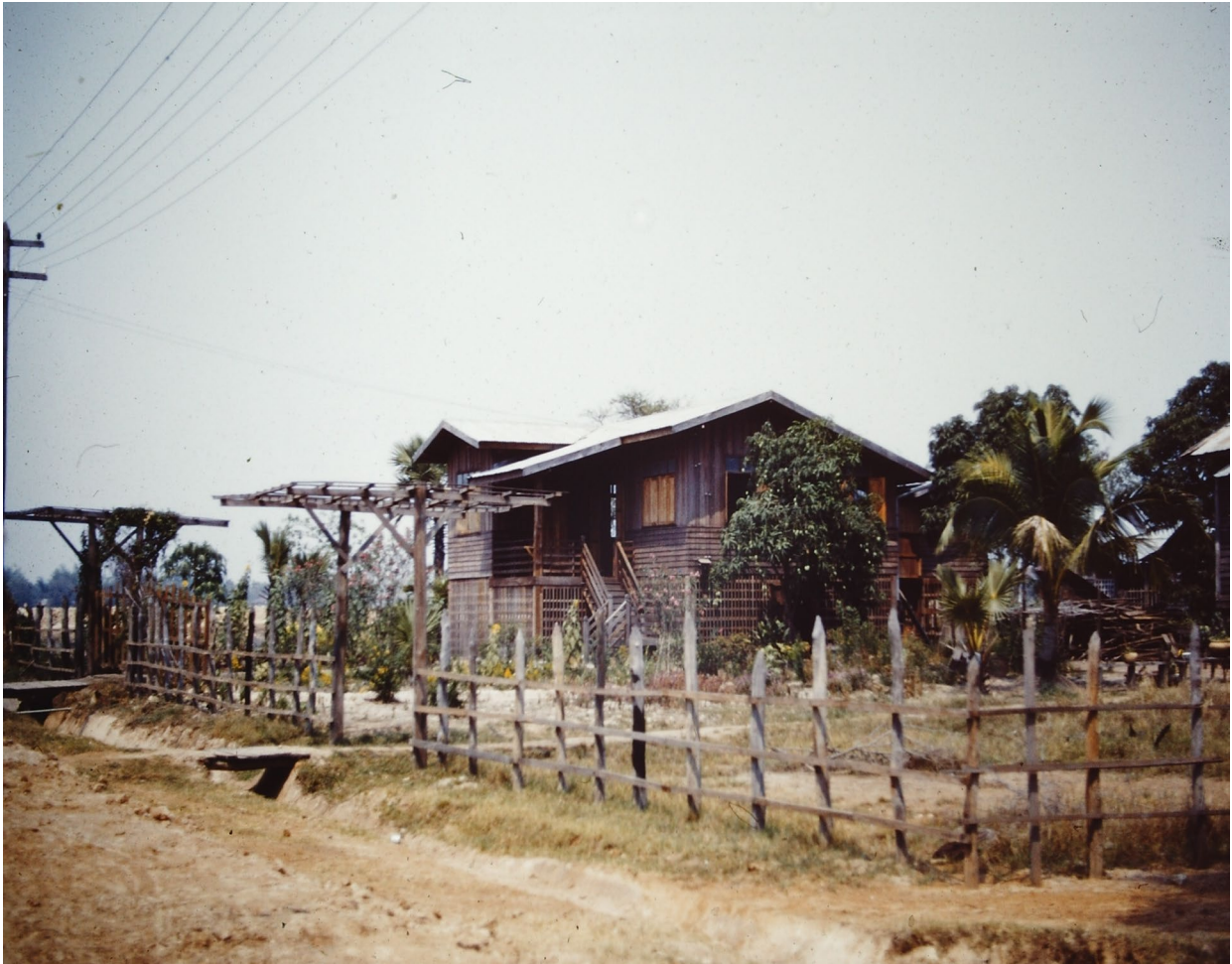
A typical raised Thai house constructed of wood and a corrugated tin roof. This particular house, located across the street from the airbase, was later rented by CJ Abadie.
