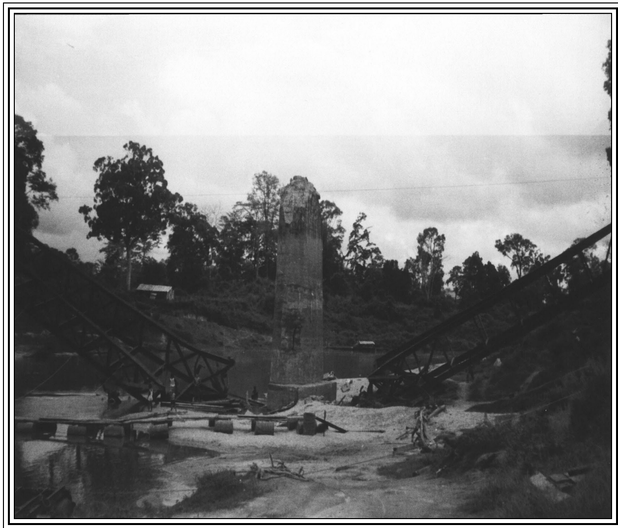
Destroyed French bridge at the Nam Lik river crossing. A rude, damaged empty fifty-five-gallon drum pontoon foot bridge floats in front of the main bridge.
