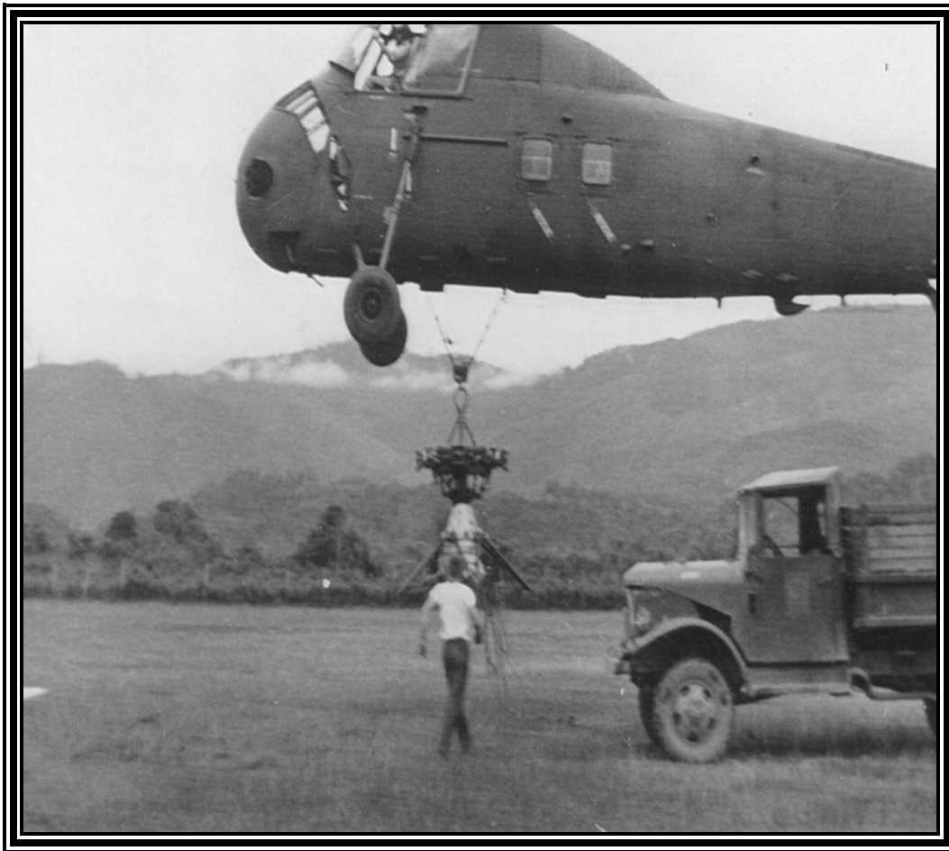
An H-34 crew delivering a quick change rotorhead and transmission to Vang Vieng for a field installation.
