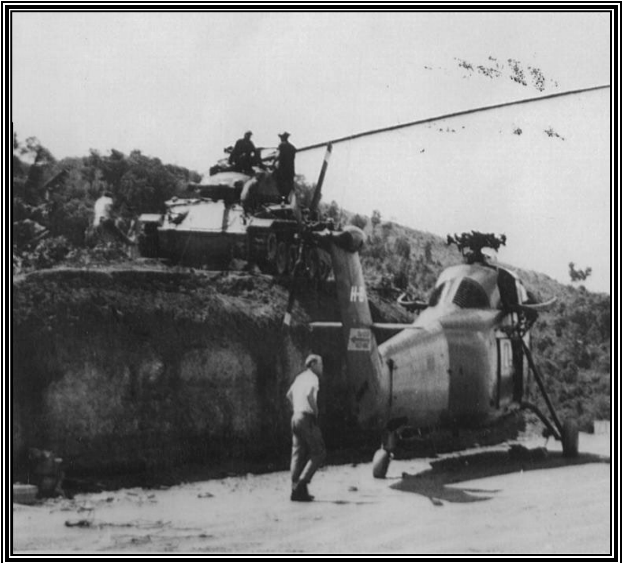
Hotel Bravo rotor head repair utilizing initiative—a U.S. Marine Corps field expediency—a Lao tank and a stout pole.
