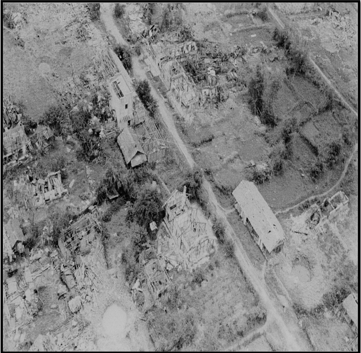
Destroyed infrastructure along Route-04 at Xieng Khouang Ville, Laos. Thompson Collection.
