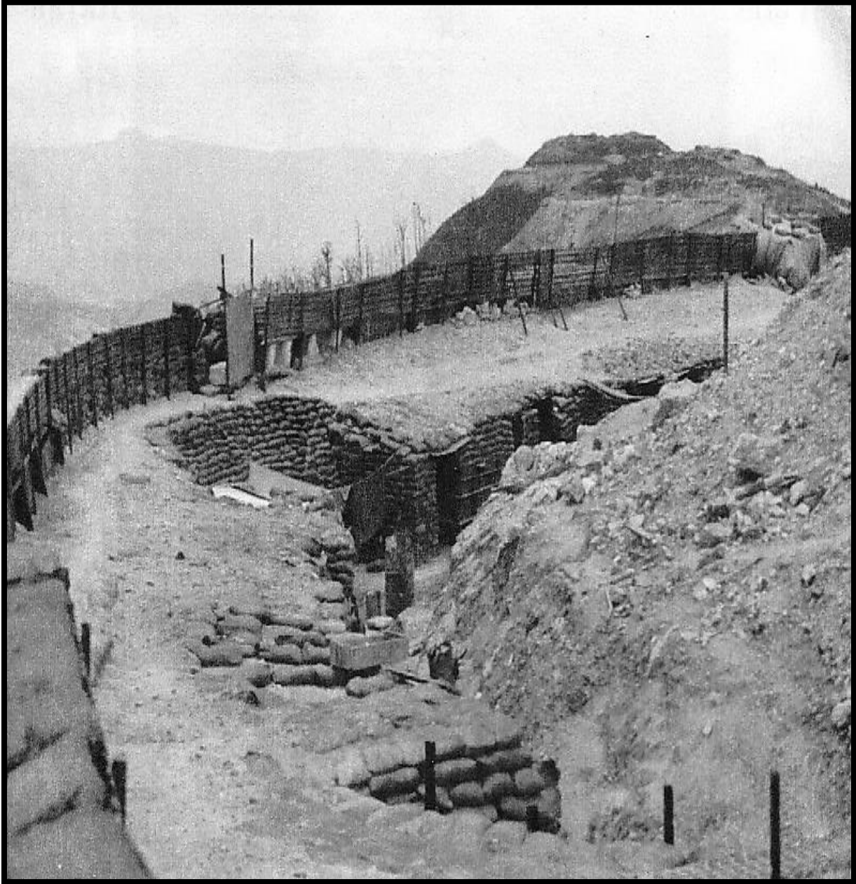
An expanded view of the previous photo showing a defensive perimeter fence, earthworks, shelters from indirect fire, and a reinforced trench line.
