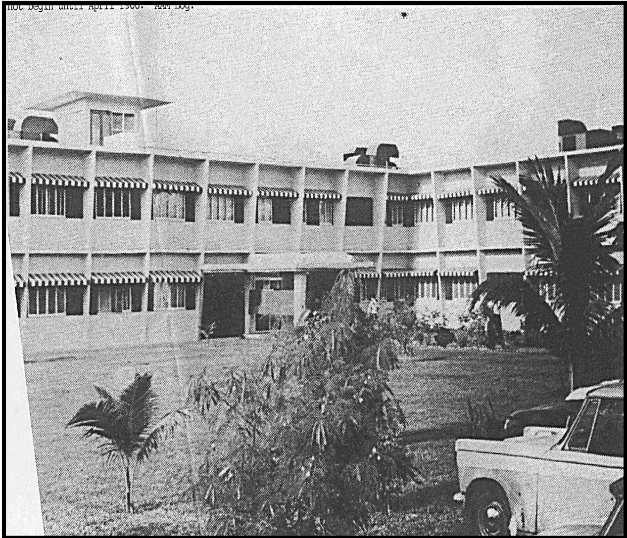
North view of Air America Udorn Administration-Operations building. Begun July 1965, construction was supervised by OICC, Bangkok. Completion and transition to the structure began during April 1966.
