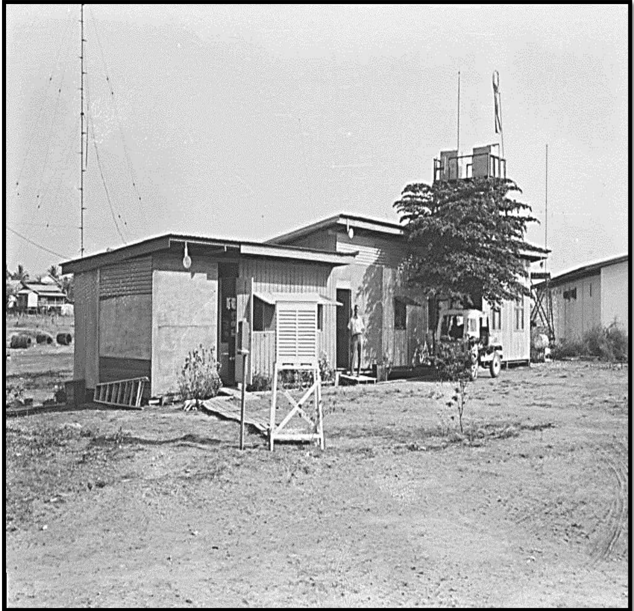
Y.C. Lueng outside the Air America radio facility Pakse, Laos. Electronic weather monitoring equipment is housed in front. Radios are contained in building to left. Personnel barracks to the right.
