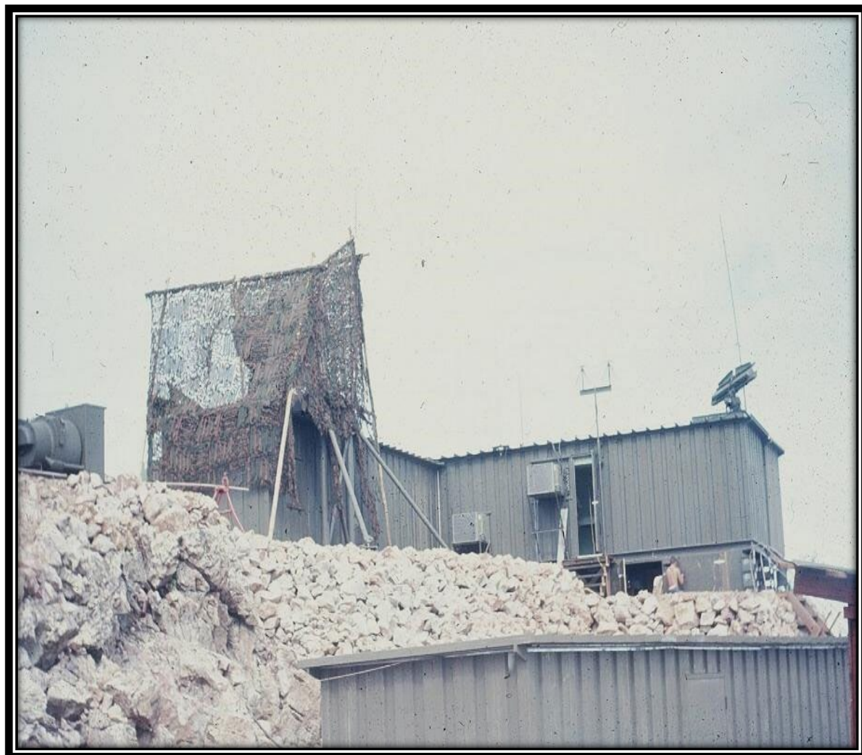
Northwest photograph of the completed TSQ-81 radar bombing control facility installed on top of Phu Pha Thi during the late summer of 1967.
