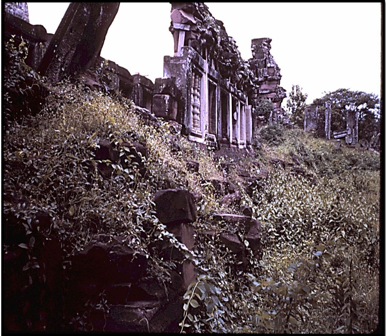
One side of the raised Pimai ruins revealing the advanced state of deterioration.
