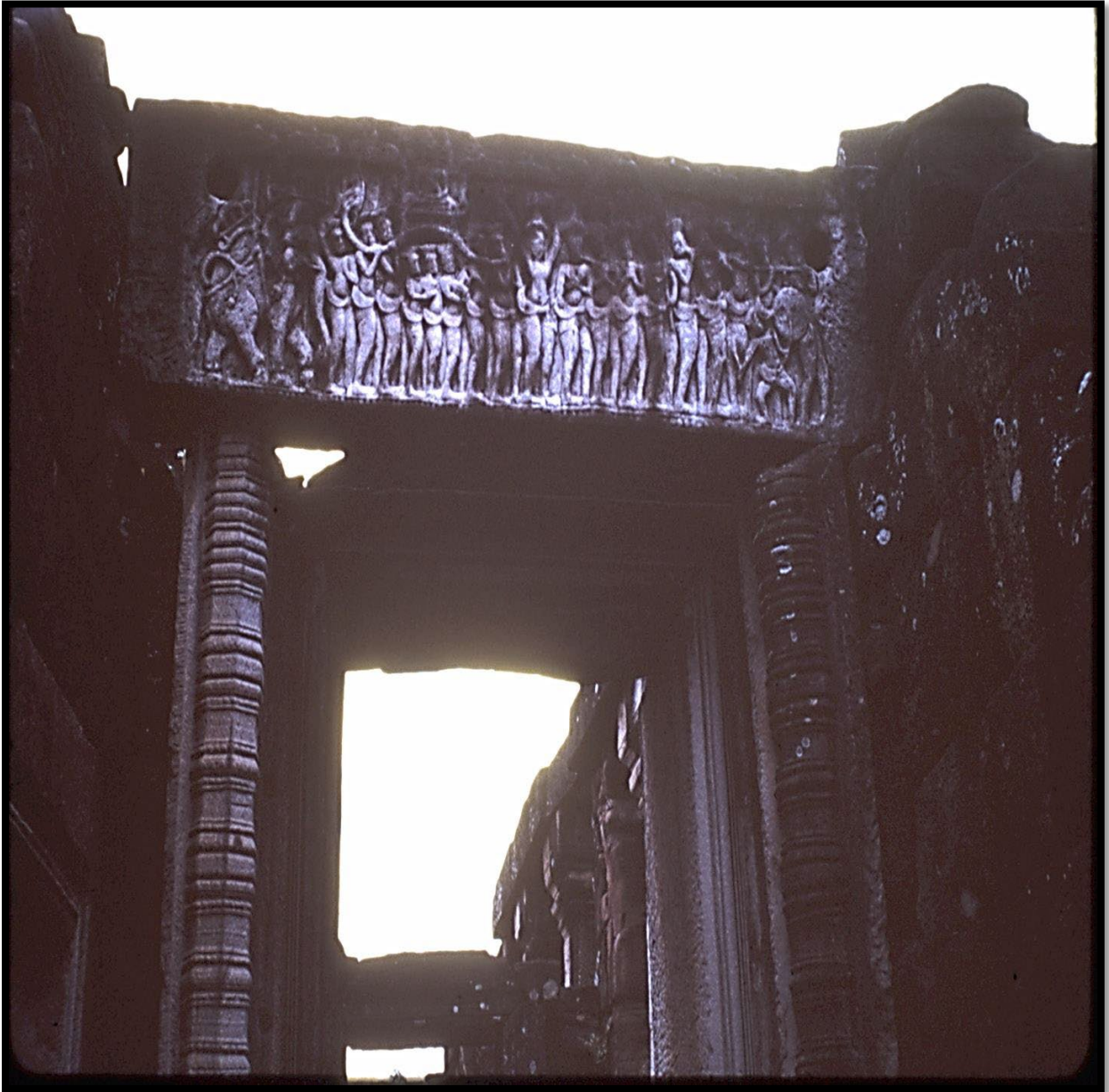
One entrance with a well-preserved lintel of story-telling images in bas-relief.
