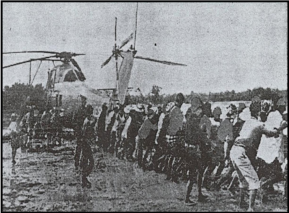
Local Thai villagers were engaged to pull EM-47 to drier ground to permit a field engine change.
