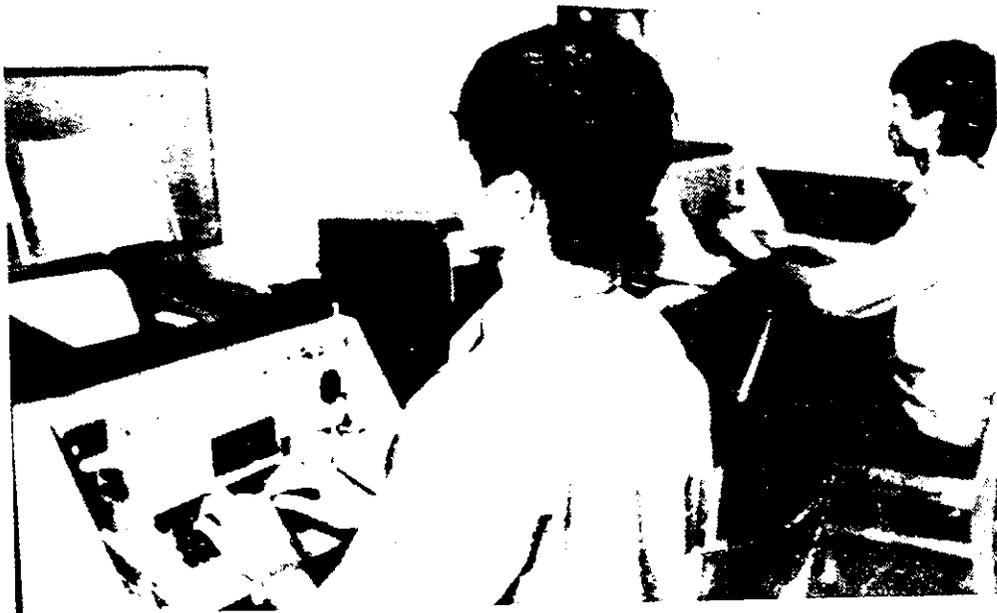
**Cipher machine use in the Air Force Service Crypto Bureau**
